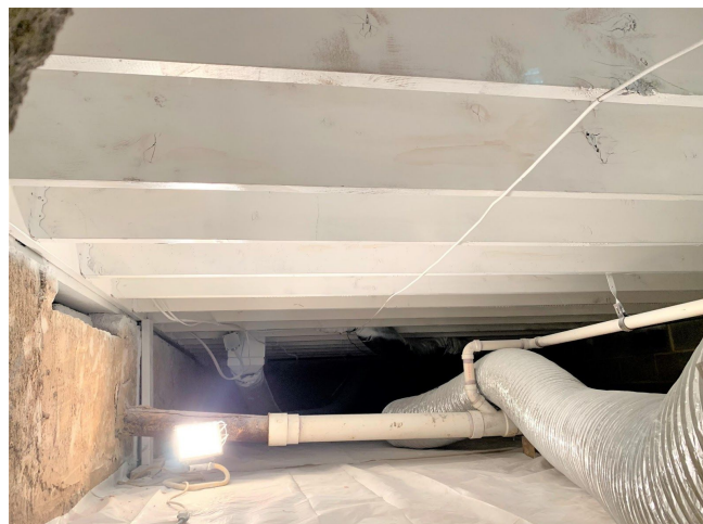
Crawlspace No. 2 - Before & After mold remediation and application of white mold-proof coating.
