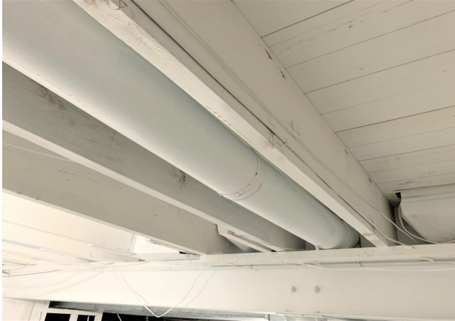
Basement Ceiling after suspended ceiling removal, surface mold remediation and application of white mold-proof coating.
