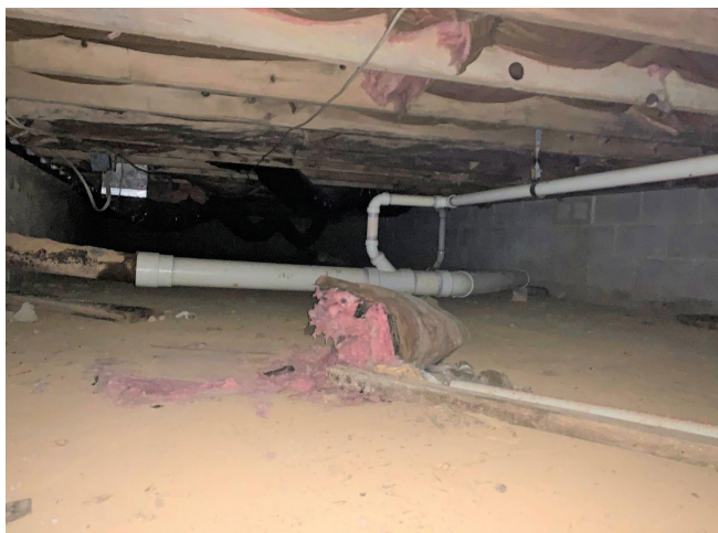
Crawlspace No. 2 - Before & After mold remediation and application of white mold-proof coating.
