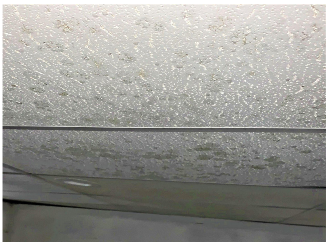
Visible mold growth observed on Basement ceiling tiles, joists, and subfloor before remediation.
