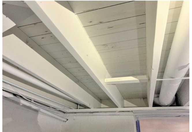
Basement Ceiling after suspended ceiling removal, surface mold remediation and application of white mold-proof coating.
