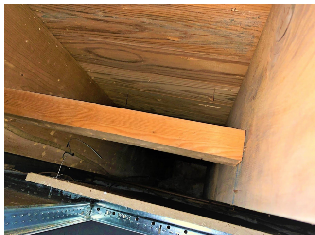
Visible mold growth observed on Basement ceiling tiles, joists, and subfloor before remediation.
