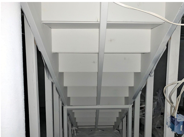
Backside of Basement stairs after remediation.
